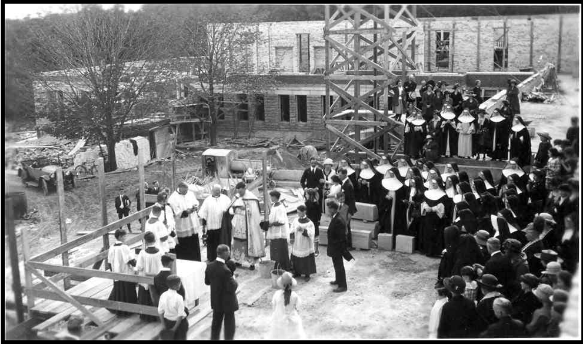
Fig. 2.1. Corner laying ceremony. Marywood Motherhouse, 1921. 186
