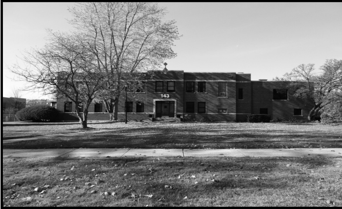
Fig. 2.3. The Lakeside Drive structure as it looks today. A two-lane road separates it from neighborhood homes. 194
