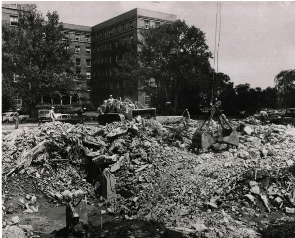
Site of demolished Gotham Hotel in 1963.
