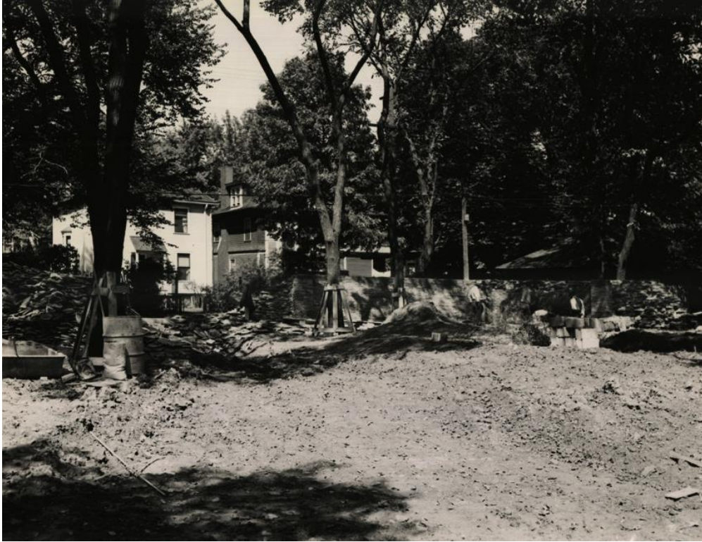
235 Holbrook - site of Roxborough's mansion being built in 1936.
