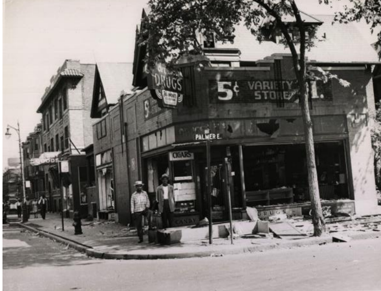
One of several stores damaged in the Black Bottoms after the 1943 riots.
