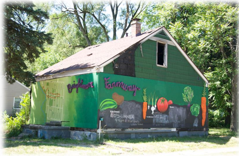
FIGURE: 5.4 BRIGHTMOOR FARMWAY COMMUNITY HOUSE
