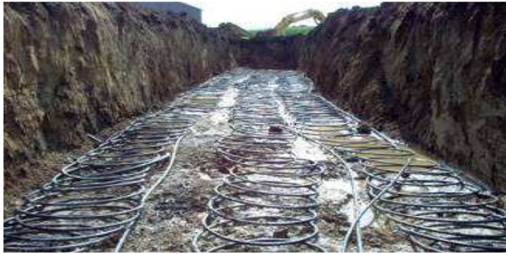
Figure 6.18: Horizontal Ground Source Heat Pump Loop
